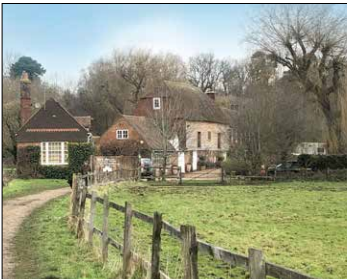
High Mill, Moor Park
