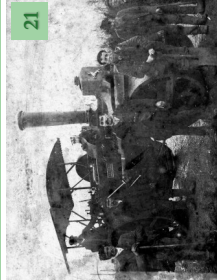
21 Workmen for Farnham Urban District Council conducting road-laying with an Aveling & Porter 10-ton steam roller c.1900 © Peeps
